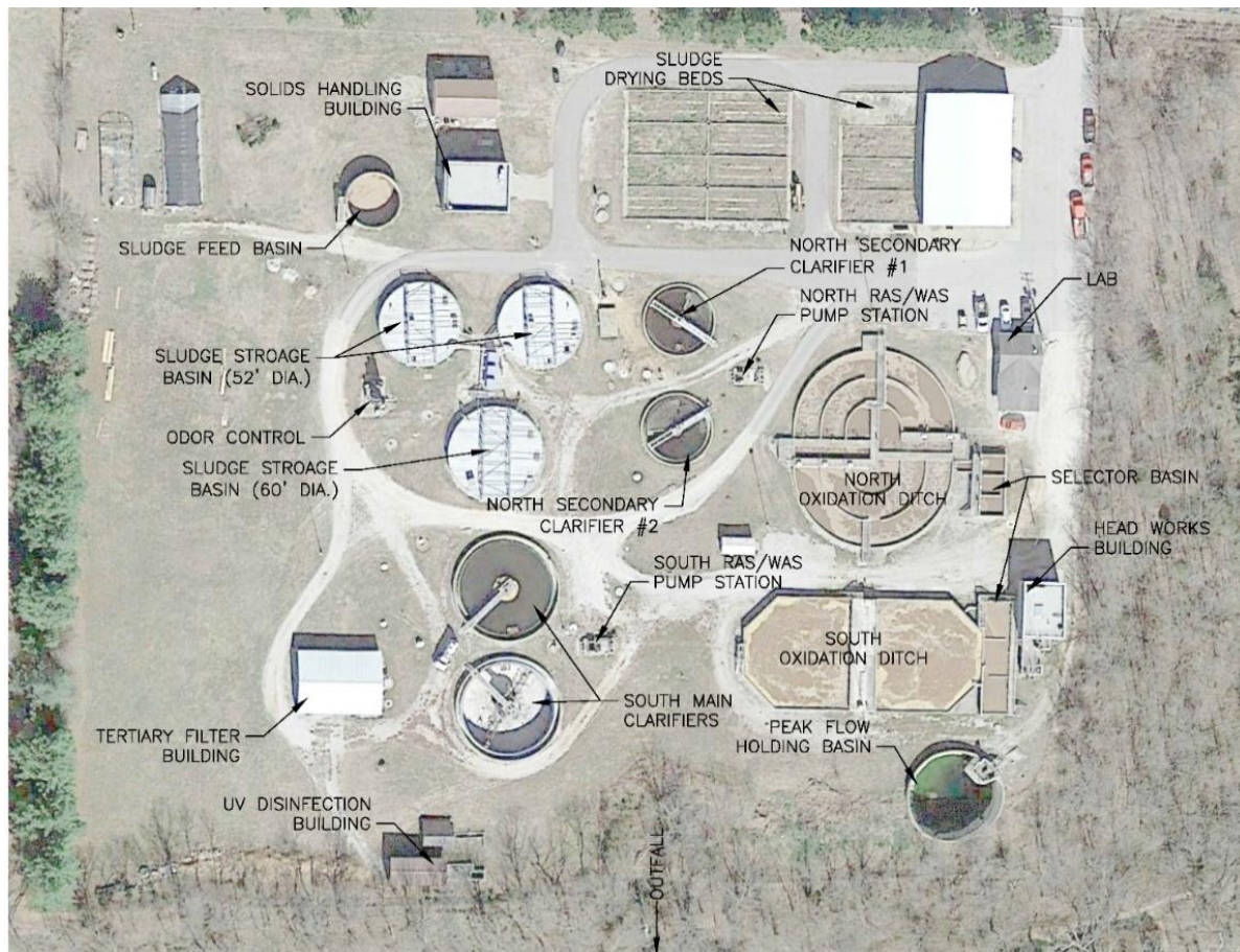
Figure 3 - Aerial Image of North 22nd Street Plant
