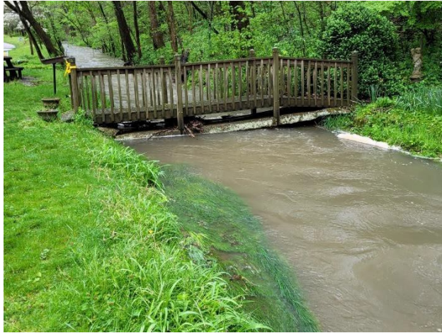
Bridge over spring branch
