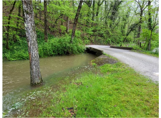
Bridge over main road culvert
