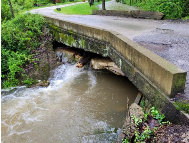
Concrete culvert on main road
