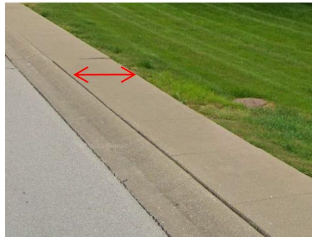
Sidewalk Cross Slope, as depicted by arrows
