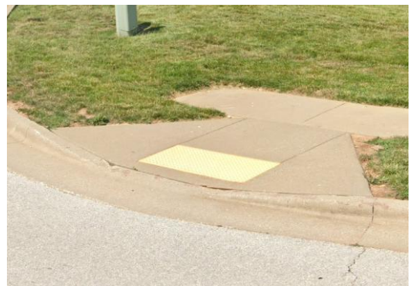
Curb Ramp Detectable Warning Surface
