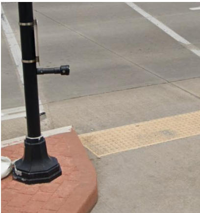
Pedestrian Signal – Pushbutton Side Reach
