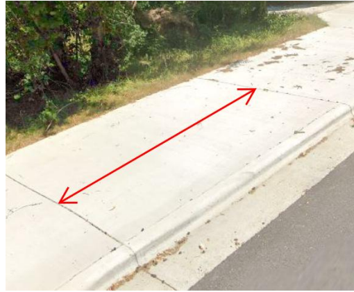
Sidewalk Run Slope, as depicted by the arrow
